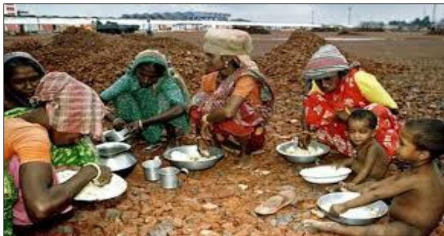
Fig 4: Women working at construction site.
